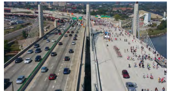
The weekend before shifting all I-95 Southbound traffic over the new southbound bridge, the community was welcomed to walk, run or bike across the main span
