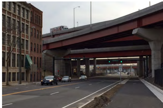
This project also included the reconstruction of 18 local roads including: East Street, Long Wharf Drive, Sargent Drive, Brewery Street and Water Street (pictured above).
